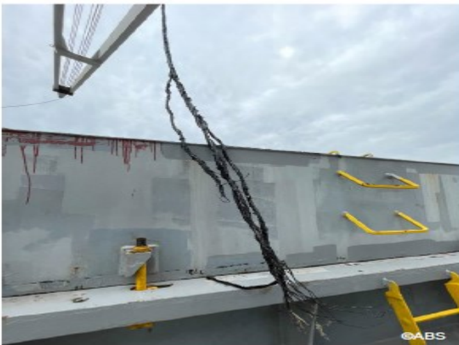
Cargo crane wire parted - before
