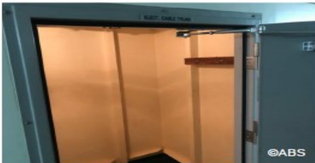
Self-closing fire door after repair
