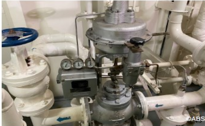
Jacket water controller cleaned after main engine propulsion control irregularity
