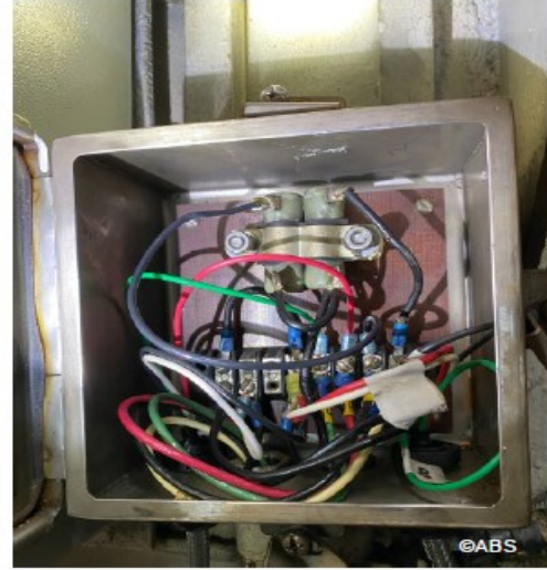
Bad connection from the transformer voltage to the power relay in the steering gear control box repaired
