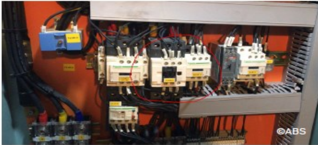
Emergency fire pump defective controller replaced
