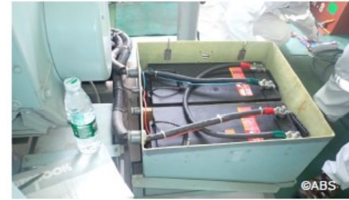
Emergency generator would not start; new batteries installed
