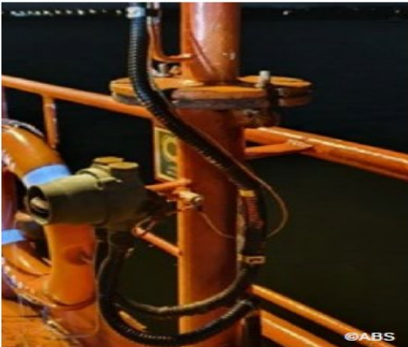
Pilot embarkation light electrical cable repaired
