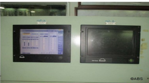
Main engine defective component for CPU replaced
