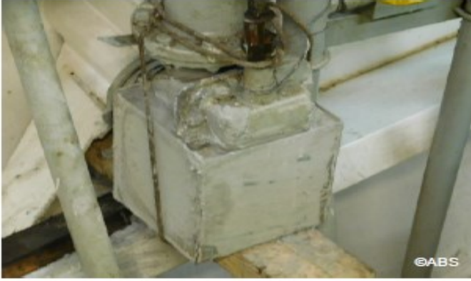
Temporary cement box repair to grey water valve
