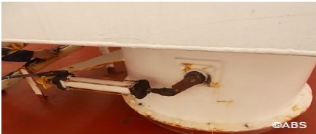
Fire damper linkage repaired
