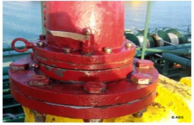
Foam monitor gasket repaired
