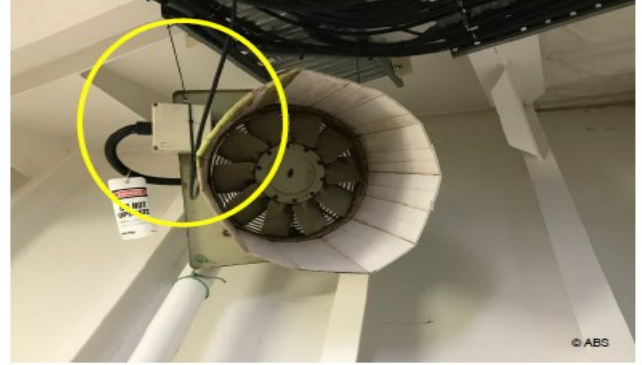
Temporary fan installed in laundry found unsafe. It was disconnected and tagged out.
