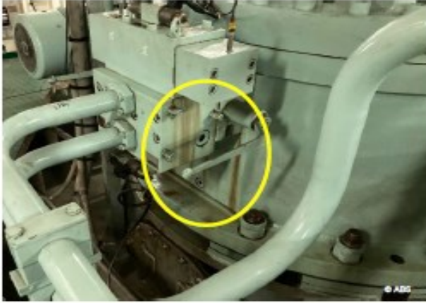
Steering gear hydraulic leaks
