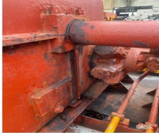
Oil leakage from winches on deck
