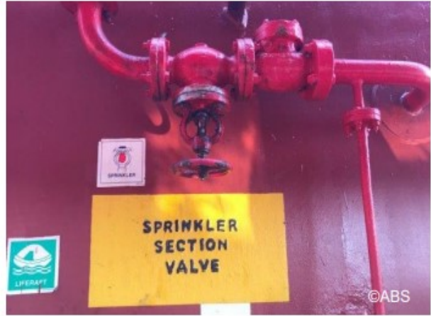
Paint room sprinkler system not in operation due to isolation valve stuck
