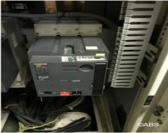
Automatic Voltage Regulator (AVR) of emergency generator malfunctioning
